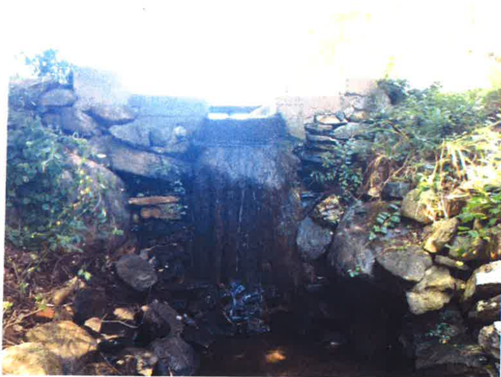
Photo 8 Downstream face of spillway
