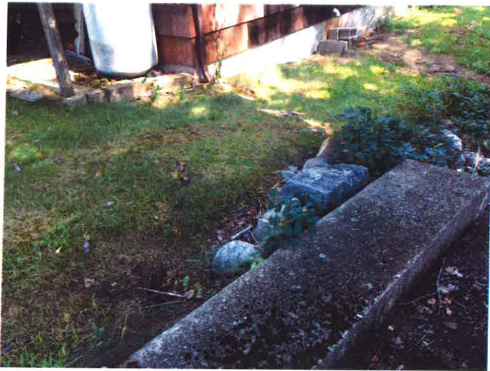
Photo 9 Erosion on left side of spillway
