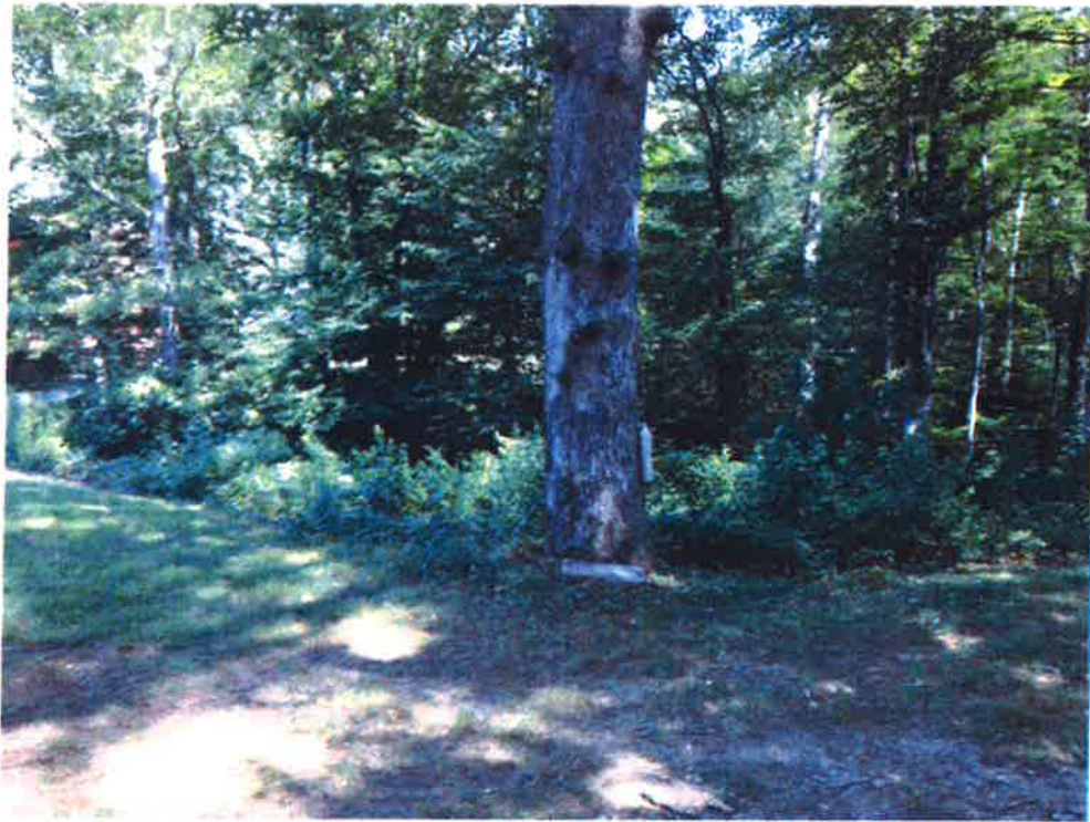
Photo 5 Large tree on downstream slope of right embankment
